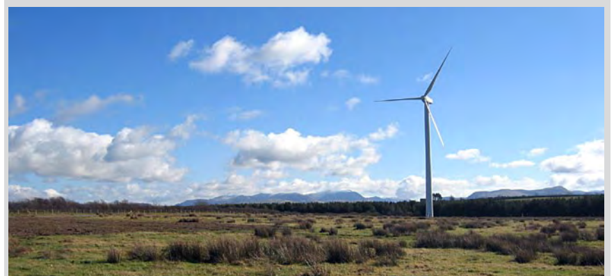
Mistral Wind has taken the reins of the now complete Winscales wind farm near Workington, Cumbria. The seven-turbine project was developed by Your Energy Ltd and features 850kW Vestas V52s. It is downwind of 11 existing turbines under the same project name but owned by Danish company KS Winscales. Photos: ERL
